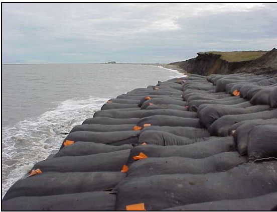
Corps Gravel Bag Revetment in 1999
